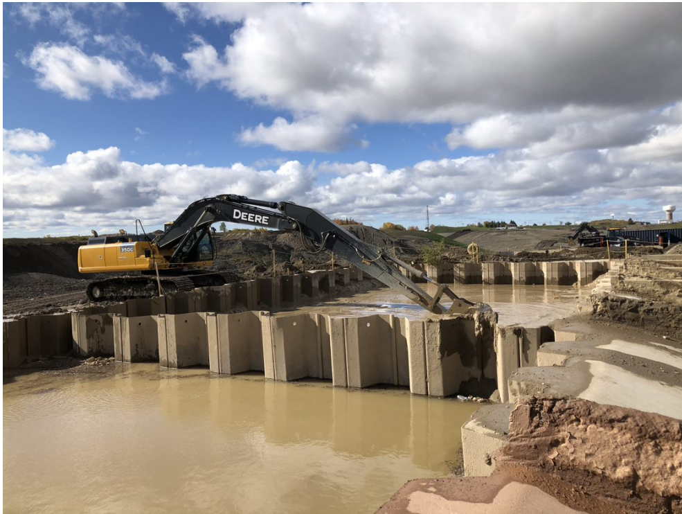
Figure v. Emptying hydrovac containment following testing.
